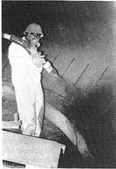
Figure 3. Shotcreting base of dome at footer location.
