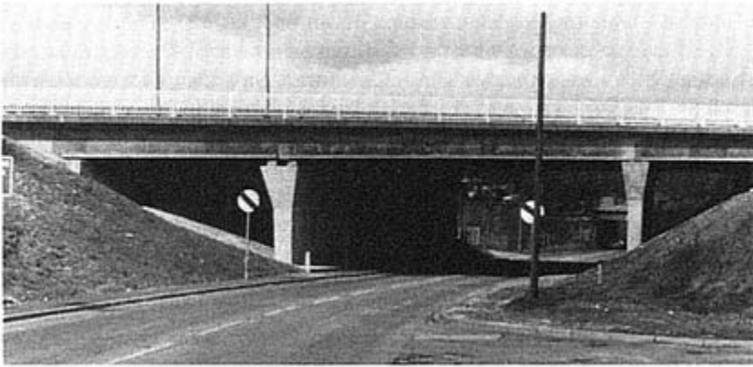
Fig. 2. View of Lawns Lane Bridge
