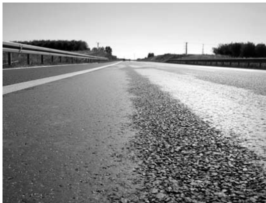
FIGURE 11.2 SMA mixture segregation—separation of mastic from coarse aggregates. (Photo courtesy of Krzysztof Błażejowski.)
