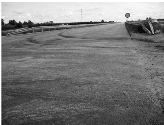
FIGURE 10.6 Soiling of an intermediate course just before laying an SMA mixture. (Photo courtesy of Krzysztof Błazejowski.)
