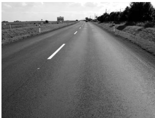
FIGURE 11.34 Mastic squeezed-out of SMA in wheel paths during trafficking of pavement. (Photo courtesy of Krzysztof Błażejowski.)
