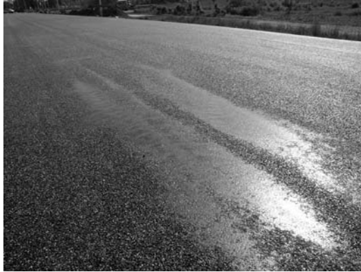
FIGURE 11.1 Longitudinal fat spots of binder. (Photo courtesy of Bartosz Wojczakowski.)
