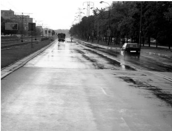
FIGURE 12.9 Differences in pavement abilities to discharge water—the SMA course ( near ) and the old dense asphalt concrete ( far ). The light reflection off the wet SMA course is substantially less than that off the asphalt concrete course. (Photo courtesy of Krzysztof Błażejowski.)
