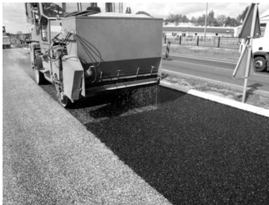
FIGURE 10.15 SMA gritters installed on rollers—the gap gritter. (Photo courtesy of Bartosz Wojczakowski.)
