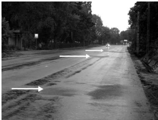
FIGURE 11.31 An example of cyclic strips of transverse porosity on a new SMA course. (Photo courtesy of Krzysztof Błażejowski.)
