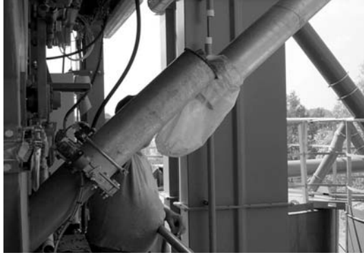
FIGURE 9.10 Performance inspection of the granulated stabilizer batching into a plant's pugmill. (Photo courtesy of Krzysztof Błażejowski.)
