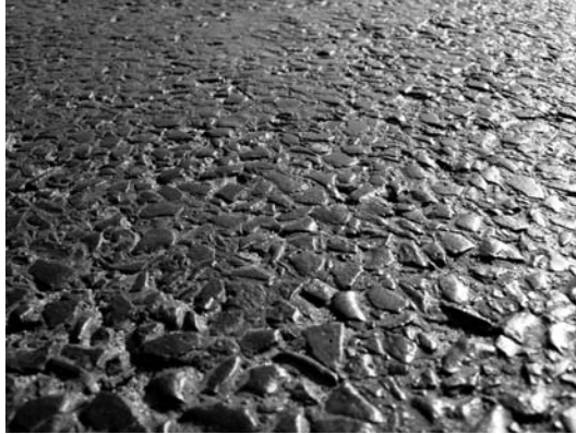
FIGURE 11.35 Polished SMA surface after 3 years of operation. (Photo courtesy of Krzysztof Błażejowski.)
