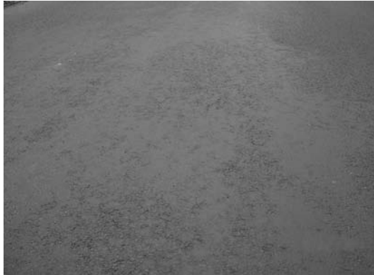
FIGURE 11.8 The closed structure of an SMA course over a large area. (Photo courtesy of Krzysztof Błazejowski.)
